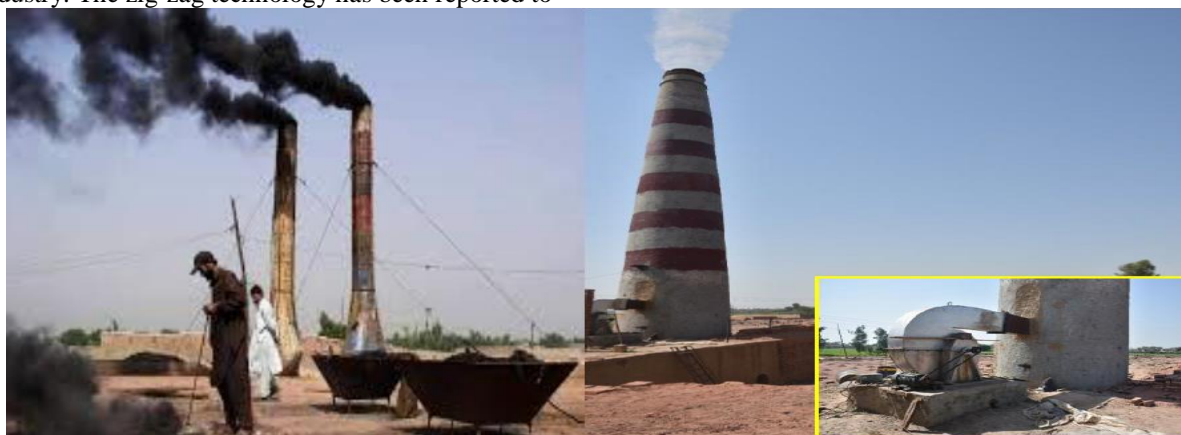
Figure 10: Old technology brick kilns vs induced draught zig-zag brick kilns in Punjab
